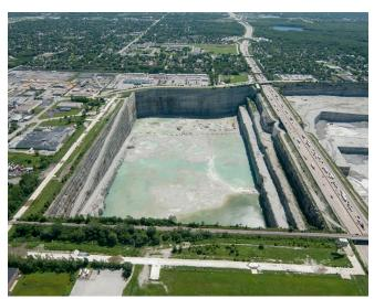
The Thornton Composite Reservoir is part of Phase II of the MWRD's TARP. The reservoir, with a volume of 7.9 billion gallons, is the largest combined sewer overflow (CSO) facility in the world. Serving a 90 square mile area in Cook County, the Reservoir provides flood relief benefits to 556,000 people in 14 communities. The project converted a limestone quarry into a CSO facility.
